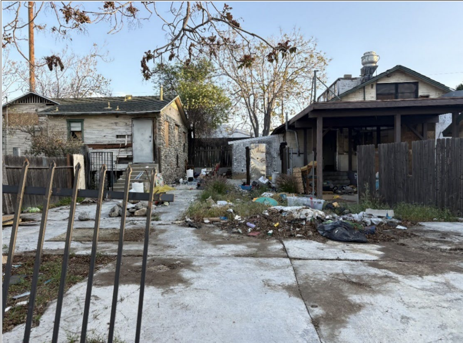
Figure 3.8 Abandoned Existing Structures
